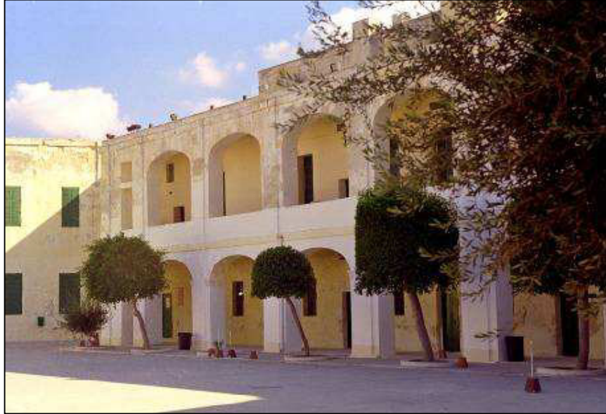
Image 3: Barrack building within Fort St. Elmo
