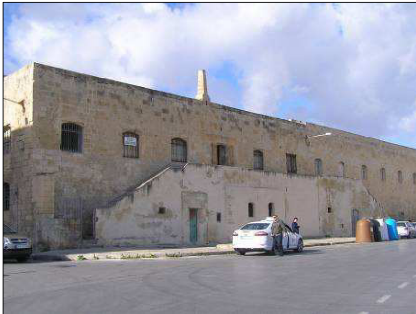
Image 14: Examination Centre front elevation
