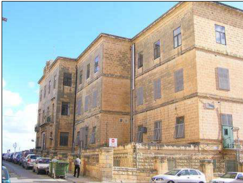
Image 12: Evans Building elevation from Triq il-Merkanti
