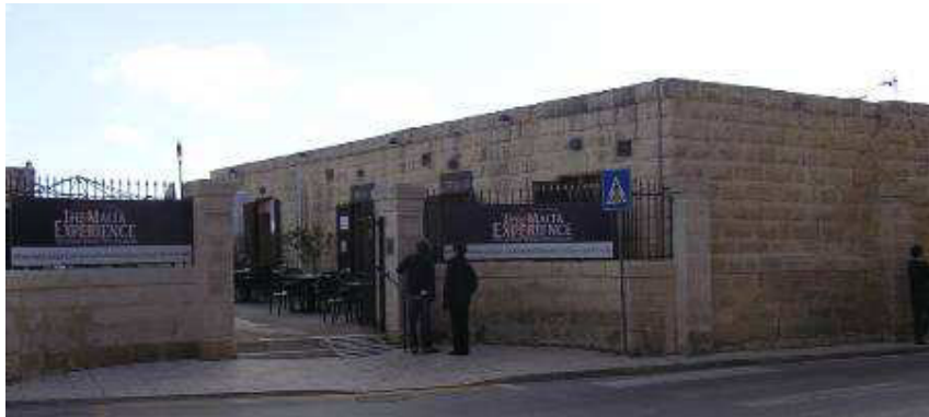
Image 9: The Malta Experience building
