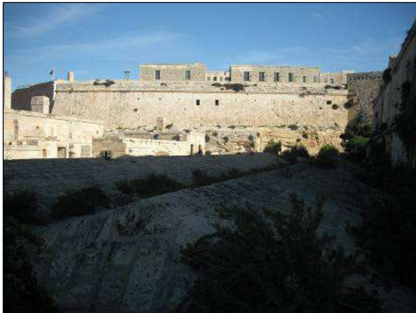
Image 6: Roof of bomb-proof Vendome water tank structures
