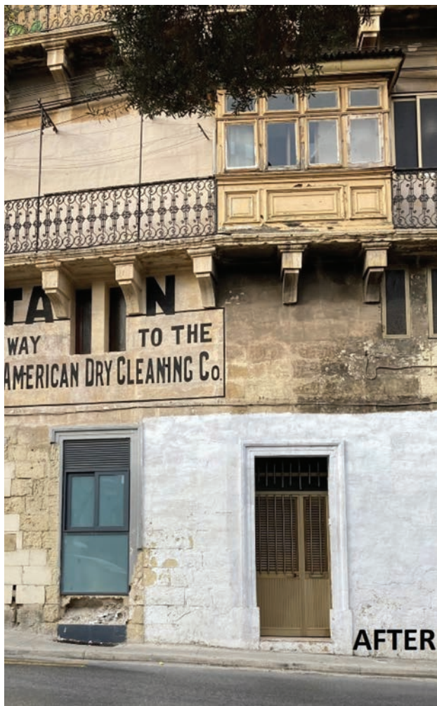
Property in Triq Il-Kbira San Ġużepp c/w Triq il-Ferrovija, Hamrun - completed restoration showing partial recovery of historic signage.
