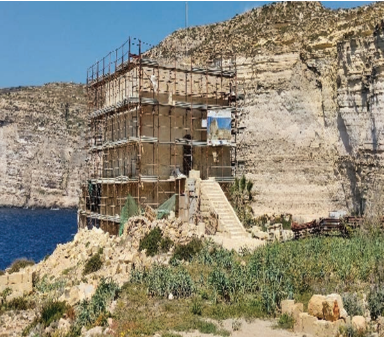
Munxar Tower – Restoration works during 2021.
