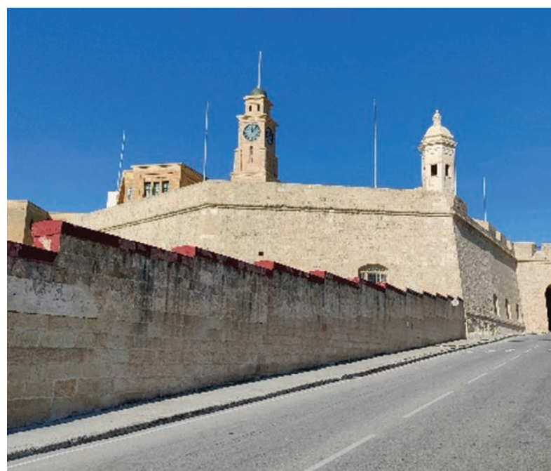
Senglea Land Front – Completed restoration works.
