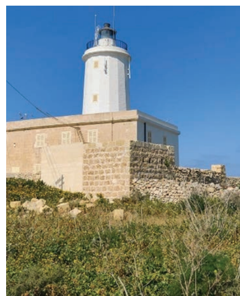
Ta' Ġordan Lighthouse - restored facades.
