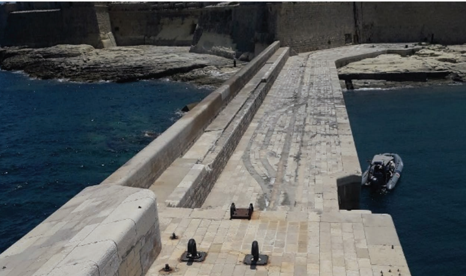
Grand Harbour Breakwater – Valletta side after restoration.
