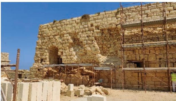
Fort Ricasoli – restoration and construction works of counterguard and casemated redoubt.
