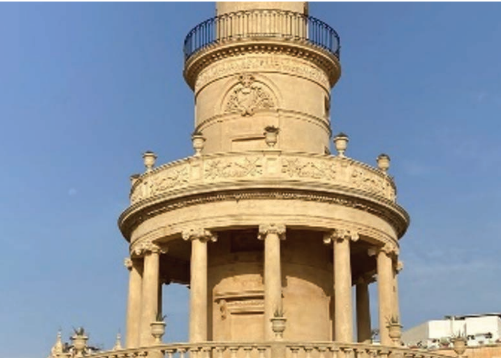
Torre Belvedere, Lija – completed restoration works.
