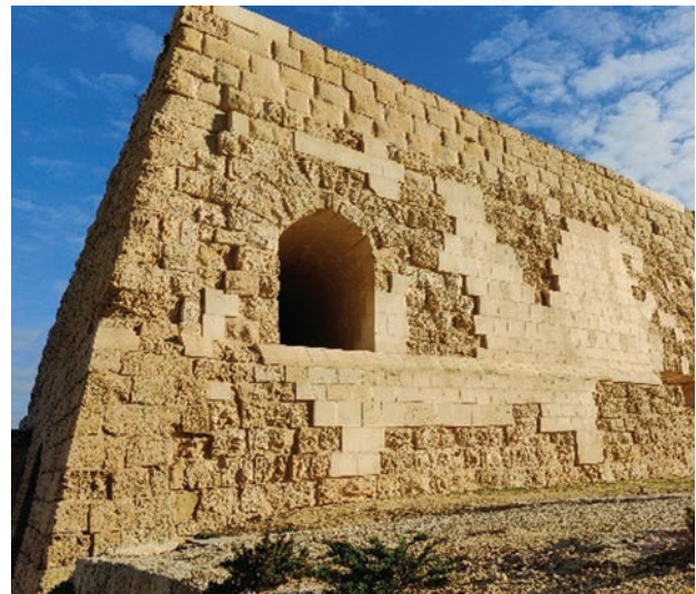
Fort Ricasoli – completed reconstruction works of counterguard and casemated redoubt.
