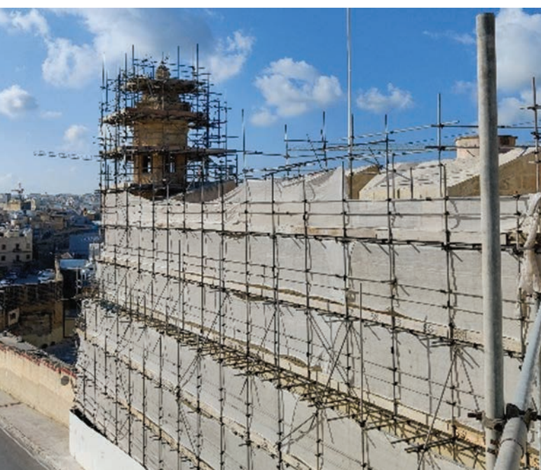
Senglea Land Front – Restoration works during 2020/2021.
