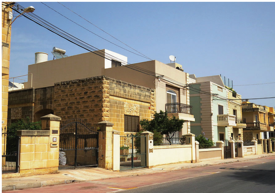
Figure 27: Well-proportioned front garden boundary walls
