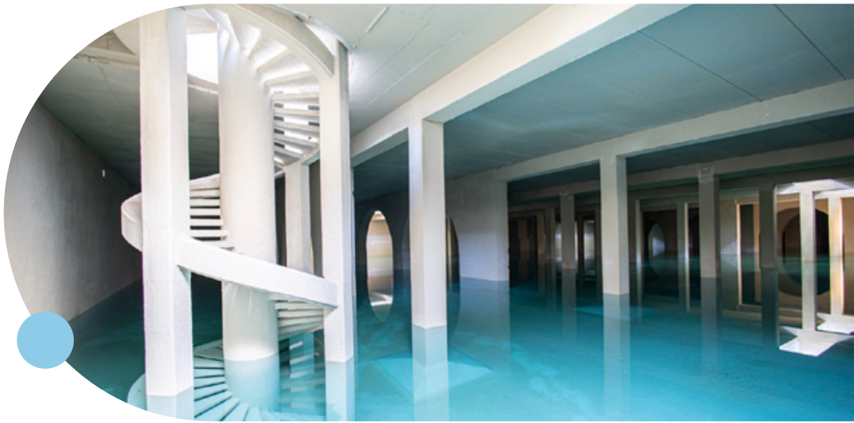
FIG Luqa reservoir filling up after major rehabilitation works .16
