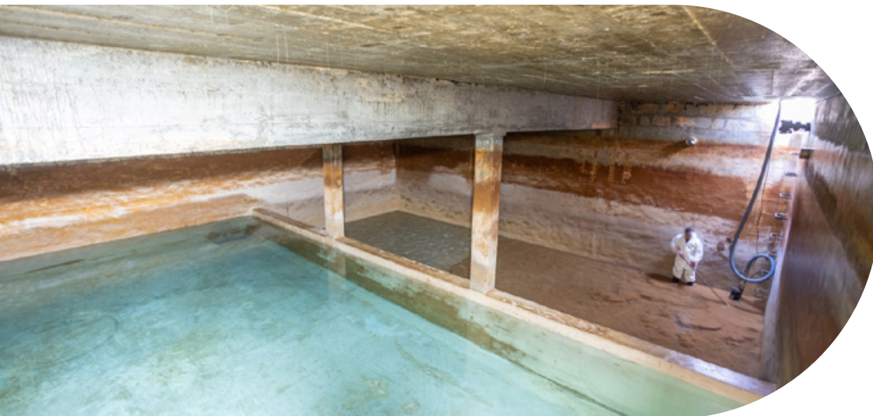
FIG Cleaning and inspection was .17 carried out at Manikata Reservoir
