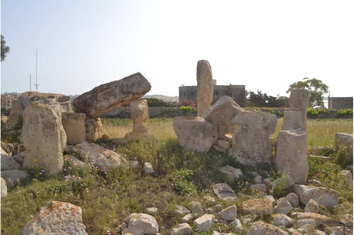
Figure 28. Photograph showing how the trilithon is resting precariously on a pillar made of modern stone blocks. Evidence of biological growth can be seen in the foreground, with weathering in the form of pitting being evident on the megalith in the left side of the photo. In the background one can observe the proximity of agricultural fields to the temple (Photo credit Josef Caruana)
