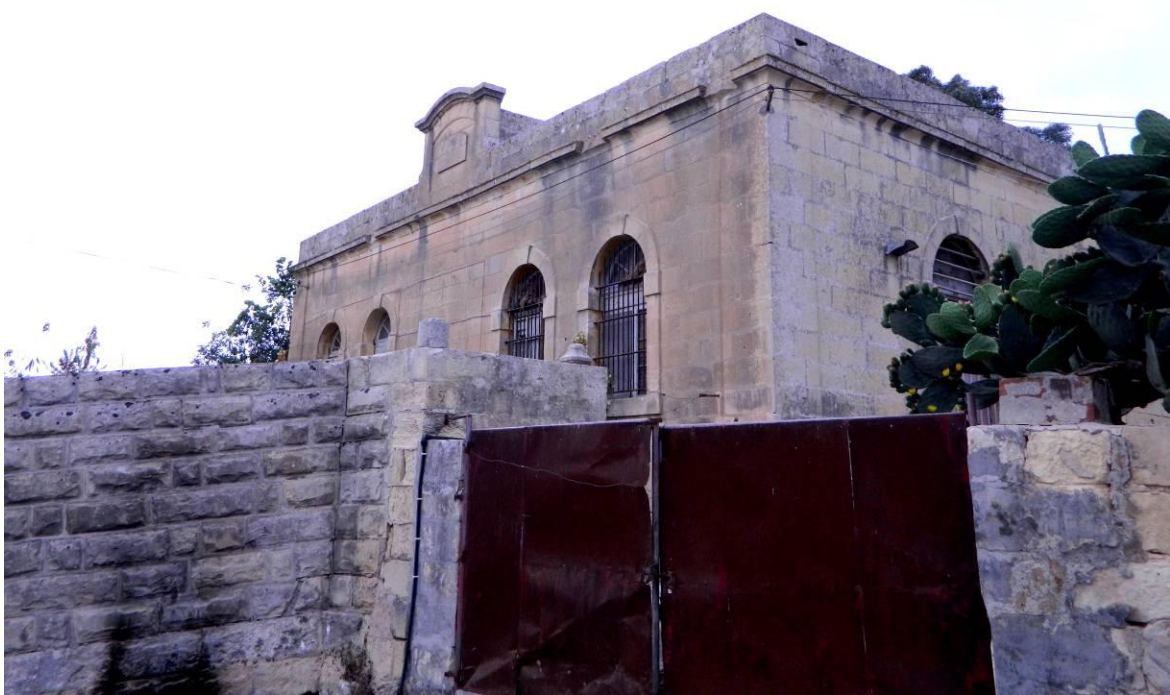
Figure 43. Pumping station at Wied Dalam (Photo credit Ruben Abela)
