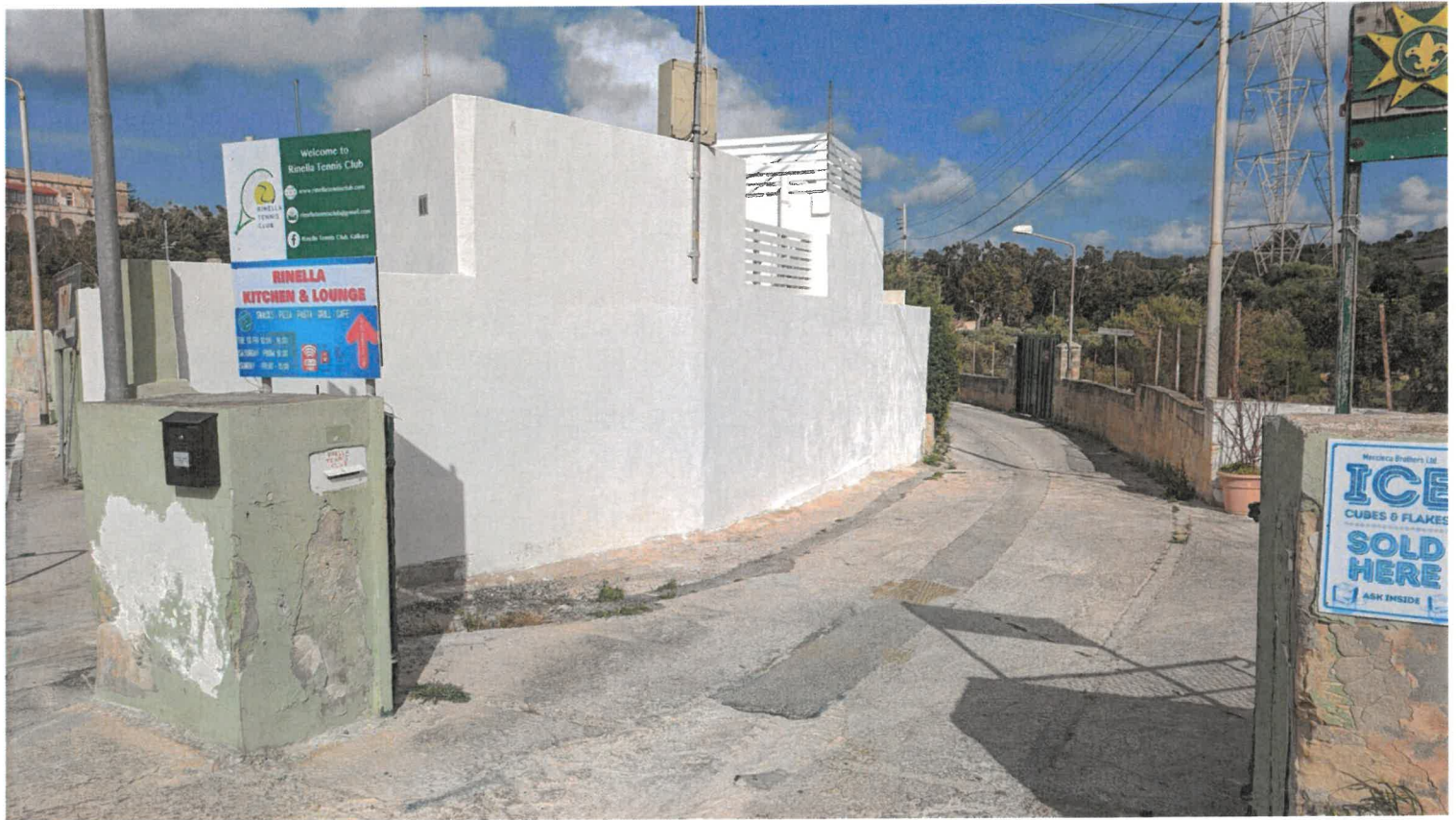
Photo 1: Rinella Tennis Pitch and facilities, Rinella (May 2023)
