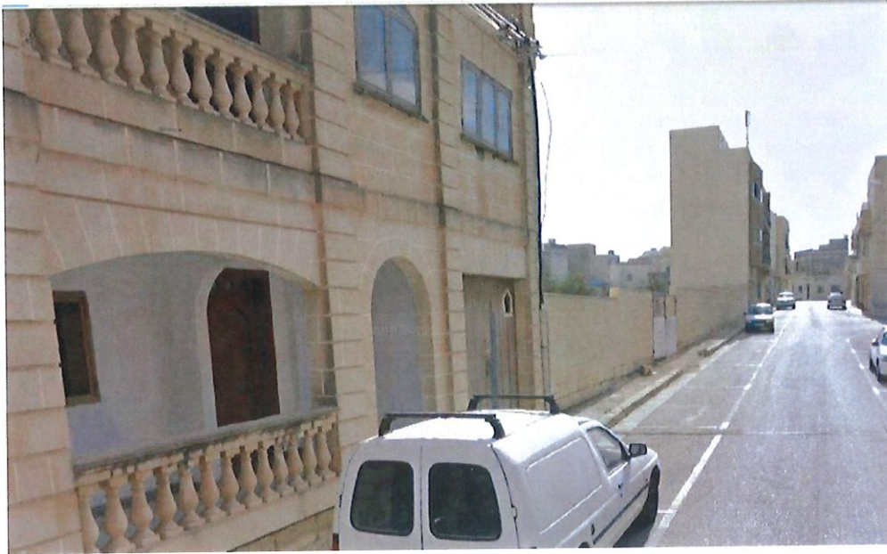
Photo 3: View of the site along Triq Salvu Sacco
