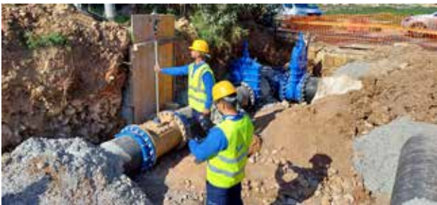
Fig. 62 Accurate location capture of network pipes and fittings
