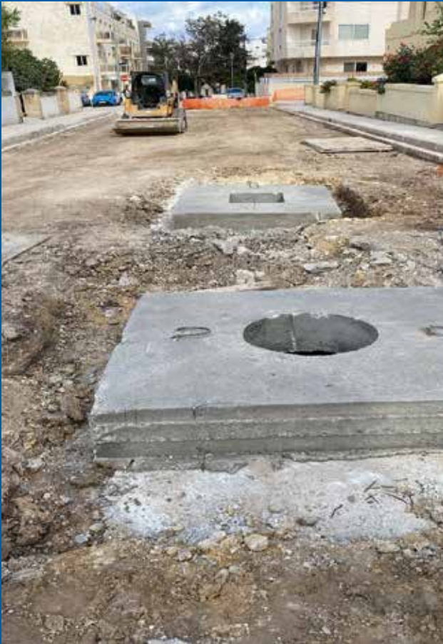
Fig. 17 Upgrades at Kalkara WWPS
