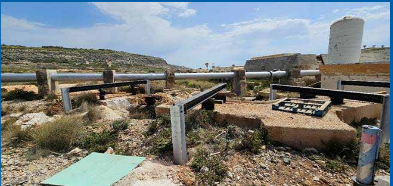
Fig. 25 Upgrading of pipework and restraining anchorage at Lapsi Reverse Osmosis plant
