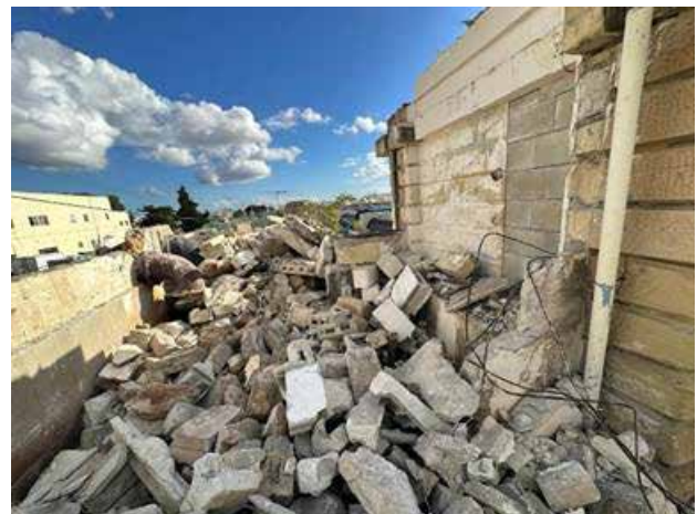
Fig. 29 Demolition of old weir room at Ta' Qali group of reservoirs
