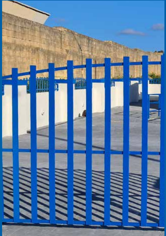
Fig. 19 Upgrades at Qajjenza WWPS
