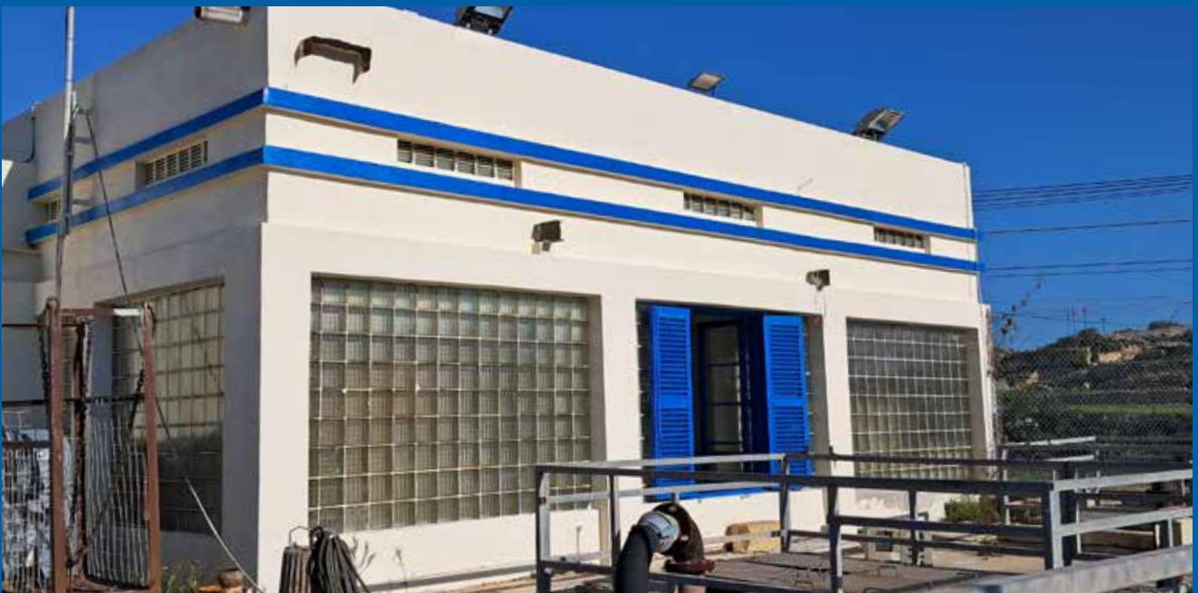
Fig. 18 Upgrades at Birżebbuġa WWPS
