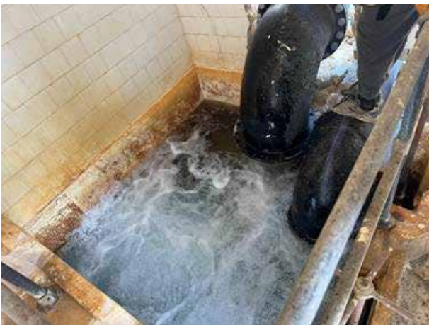
Fig. 28 Penstock chamber acting as temporary weir room.
