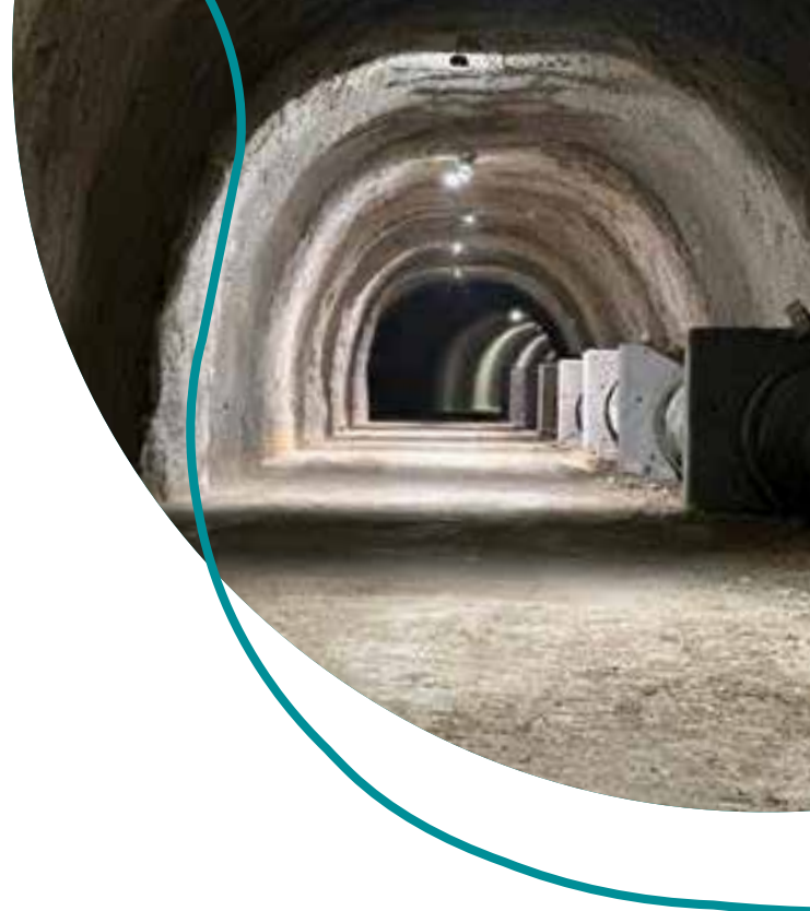
Fig. 27 The 800mm diameter pipe transporting water towards the northern harbour areas.
