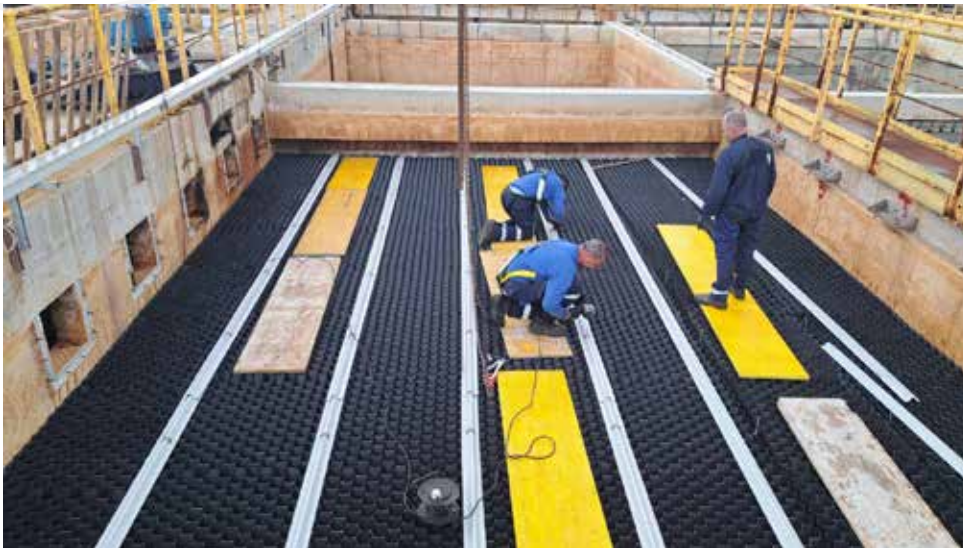
Fig. 52 Refurbishing works at the Malta South WWTP
