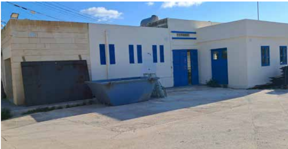
Fig. 16 Upgrades at Birżebbuġa WWPS
