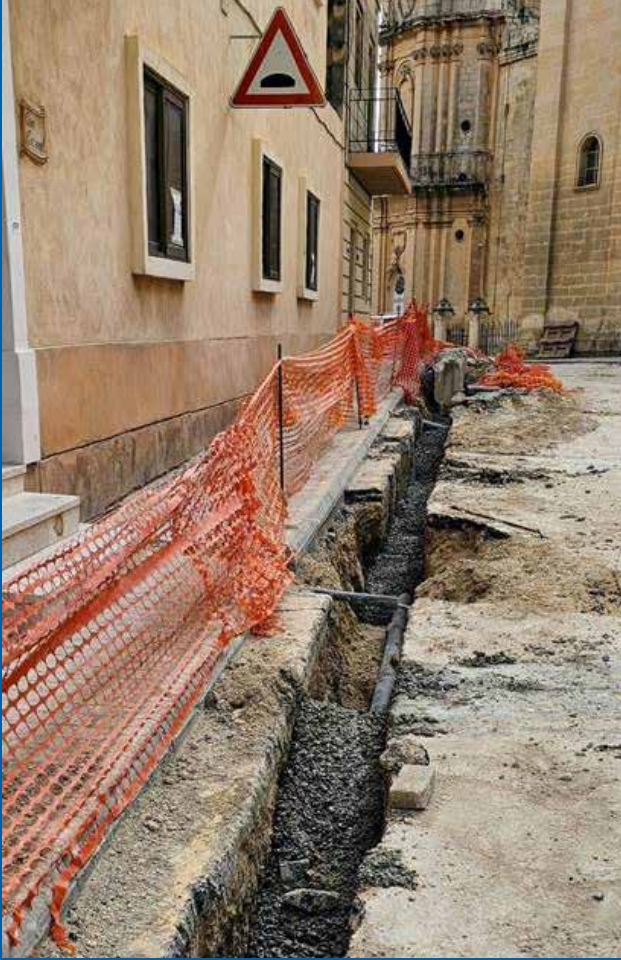
Fig. 23 Replacement of old mains
