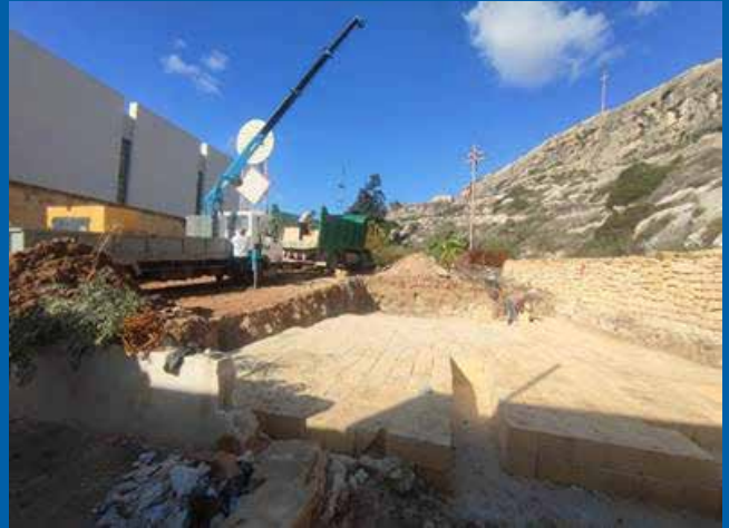
Fig. 42 Generator plinth preparation left and installation on the right
