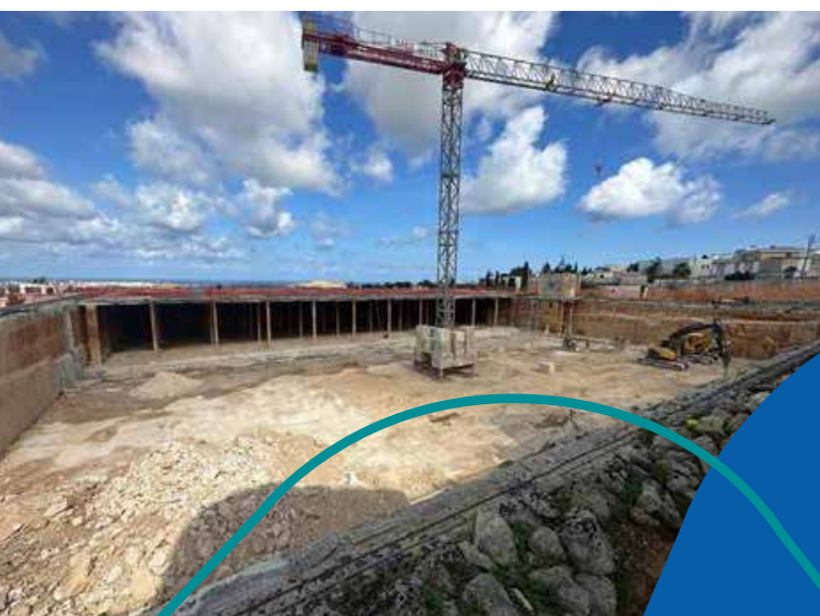
Fig. 31 Naxxar Reservoir works underway
