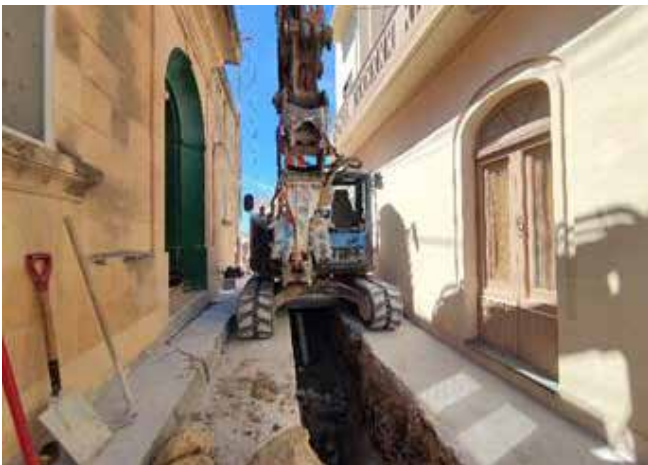
Fig. 40 General works throughout Gozo
