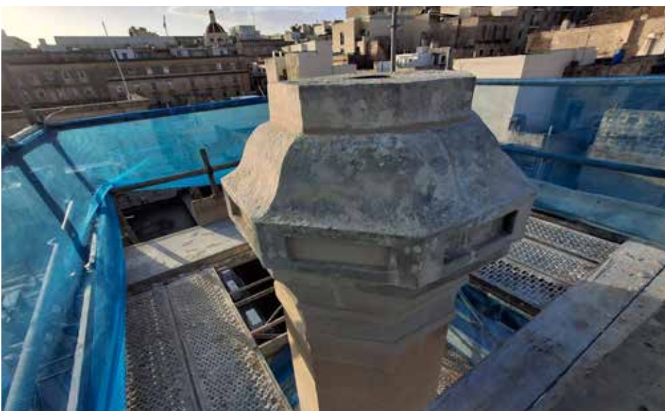
Fig. 74 The wastewater vent in Triq San Mark, Valletta, was restored
