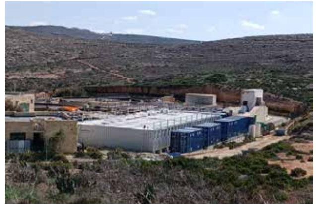
Fig. 51 Malta North WWTP
