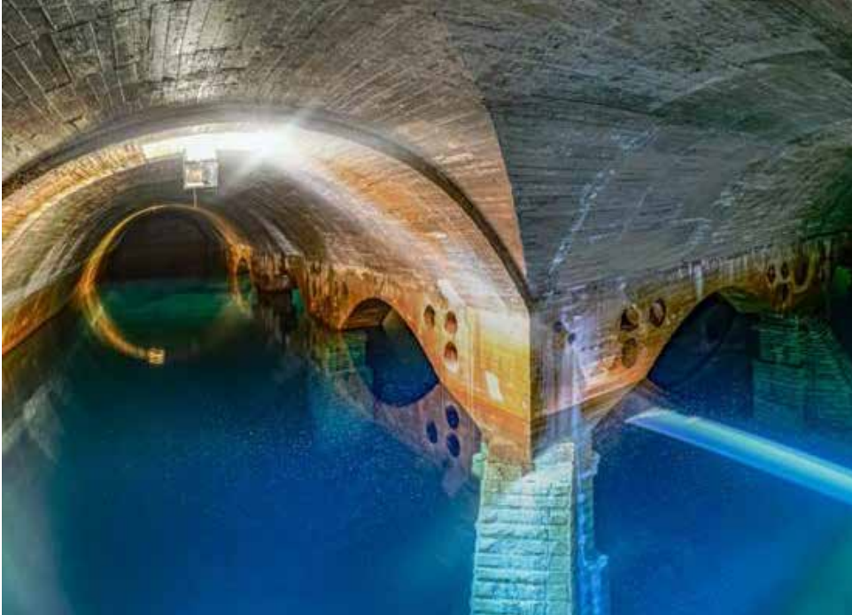
Fig. 39 Naval Reservoir during testing with 9 meters of water
