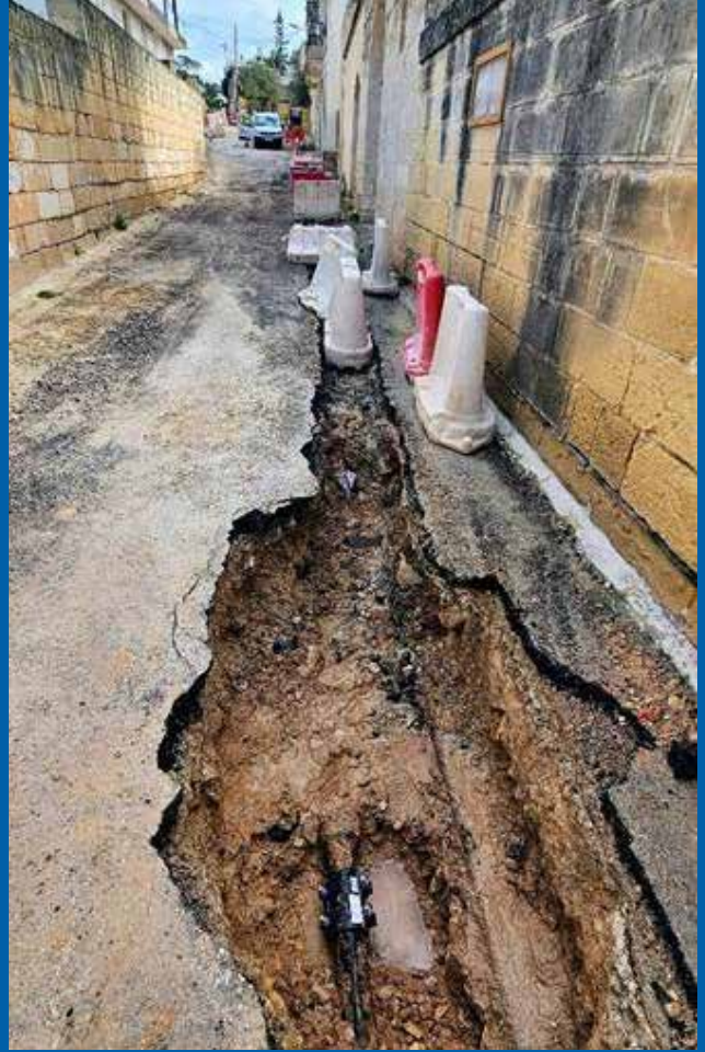
Fig. 24 Repairs carried out on mains
