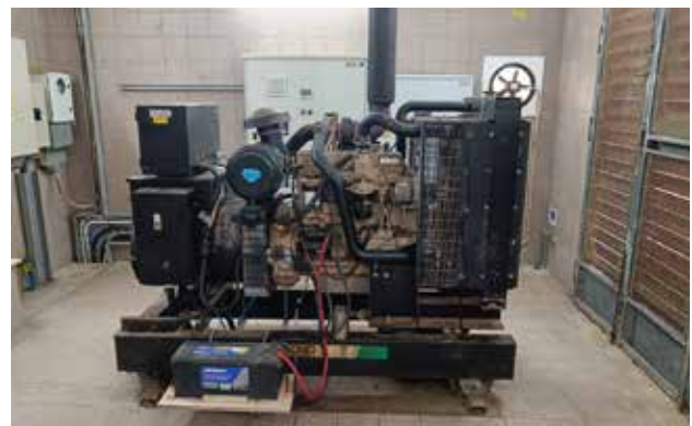
Fig. 15 New electrical control equipment at Mgarr WWPS
