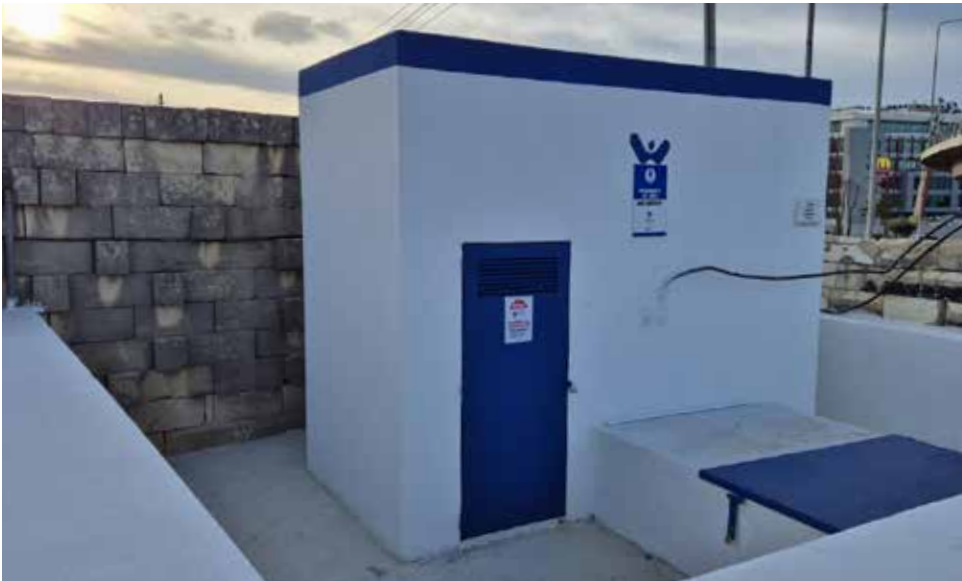
Fig. 73 Ongoing upgrades include the refurbishment of a number of WSC facilities
