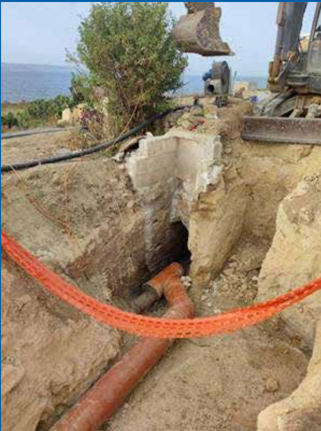
Fig. 41 Xatt L-Ahmar sewer upgrade
