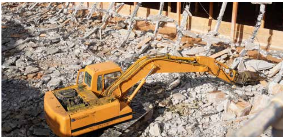
Fig. 75 Naxxar Reservoir's roof and supporting structure are being replaced
