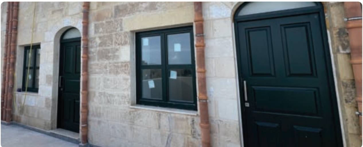
Rehabilitated Camerata Units in Valletta
