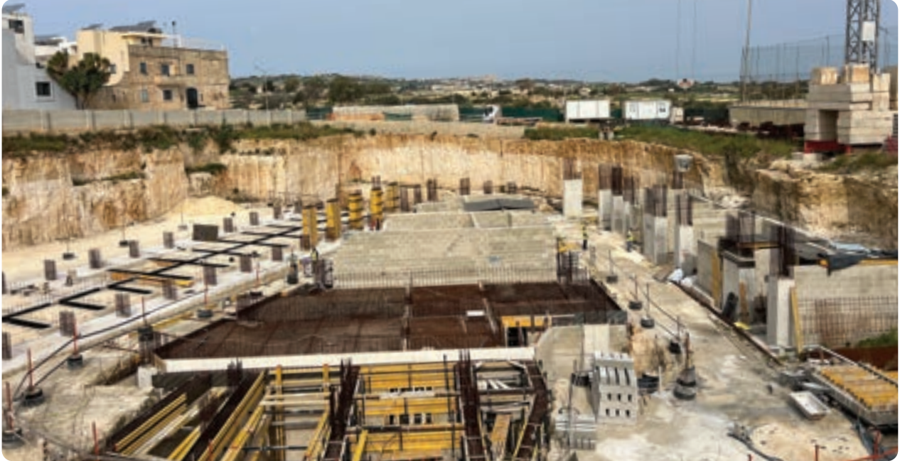
Foundation Works at Wied Hesri Complex, Siġġiewi
