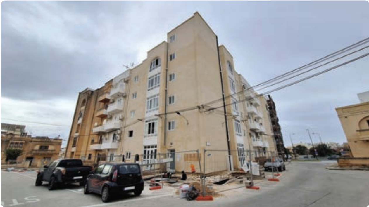
Block L, Żabbar – Deep Energy Renovation Project
