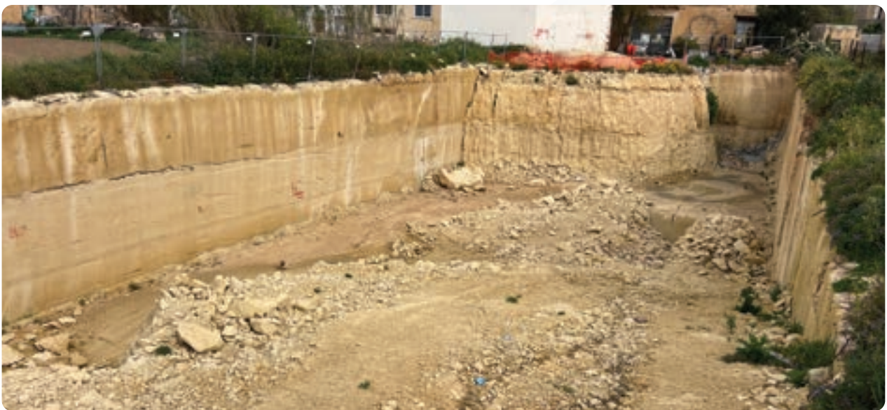
Excavation Works at Tank Street, Siġġiewi
