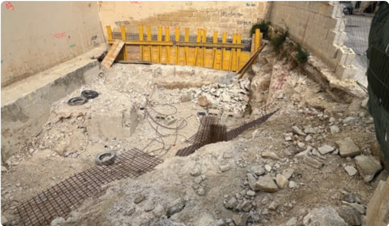
Excavation Works at S. Imbroll Street, Paola
