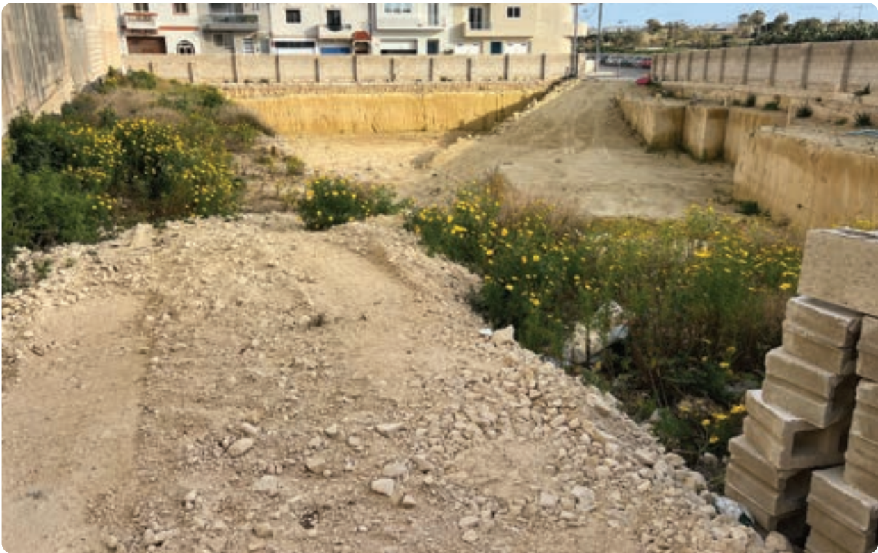
Excavation Works at Serafin Tanti Street, Żebbuġ
