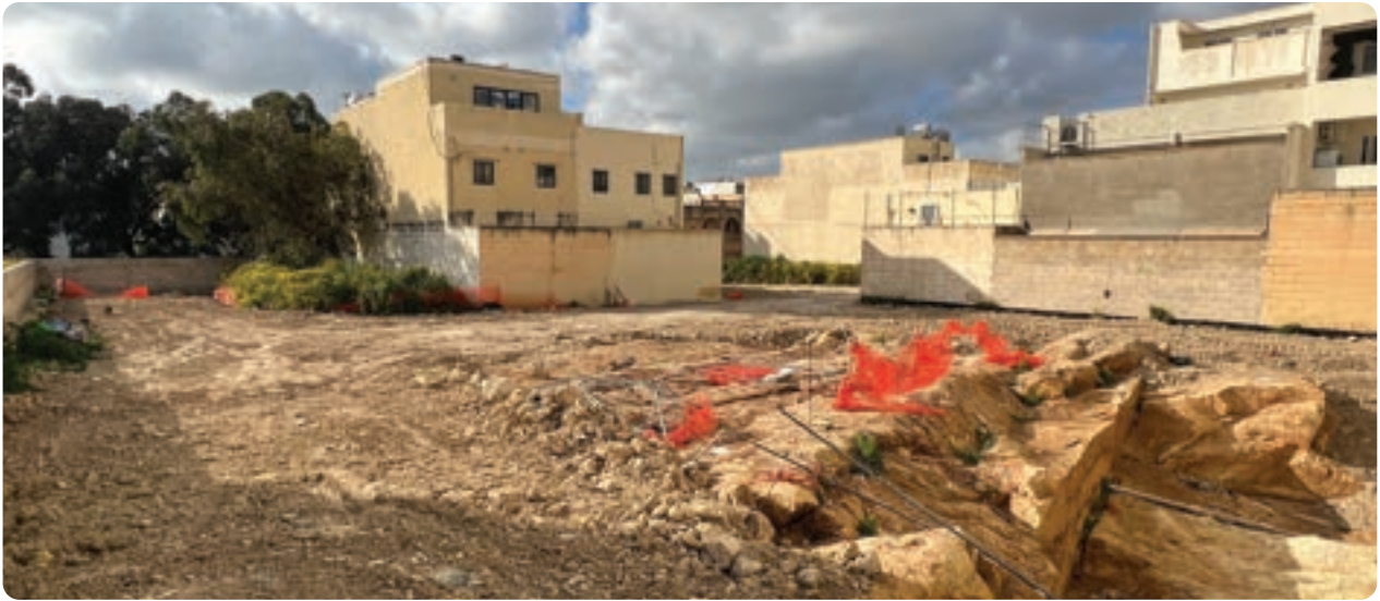
Excavation Works at Karwija Street, Kirkop
