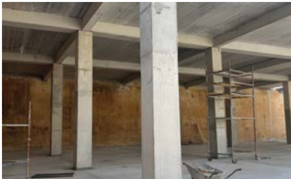
Figure 86 Naxxar Reservoir restoration
