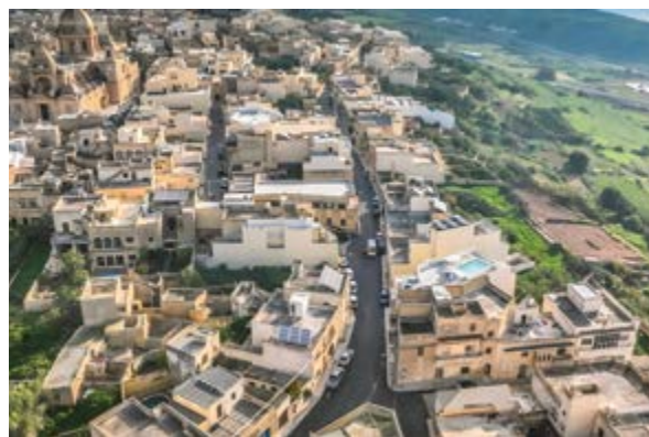
Figure 32 Extensive infrastructure replacement works in Gozo were undertaken in 2025
