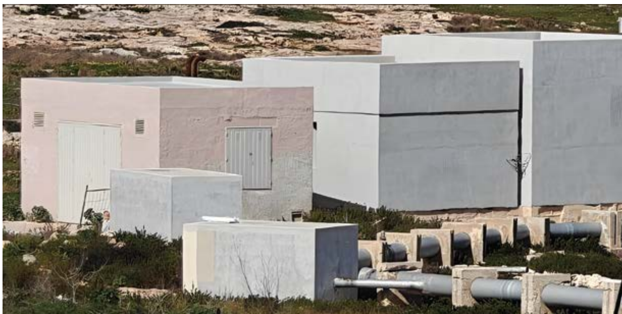
Figure 80 Rehabilitation of Pembroke well rooms
