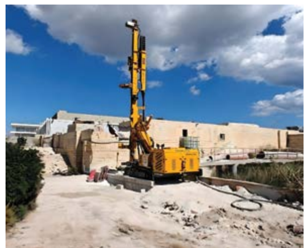
Figure 30 Drilling of seawater Borehole at Hal Far WSC site
