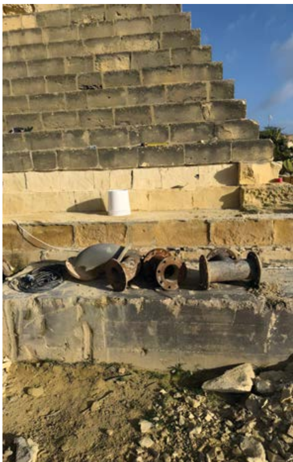
Figure 84 Ta' Ġenċ Reservoir 4 restoration
