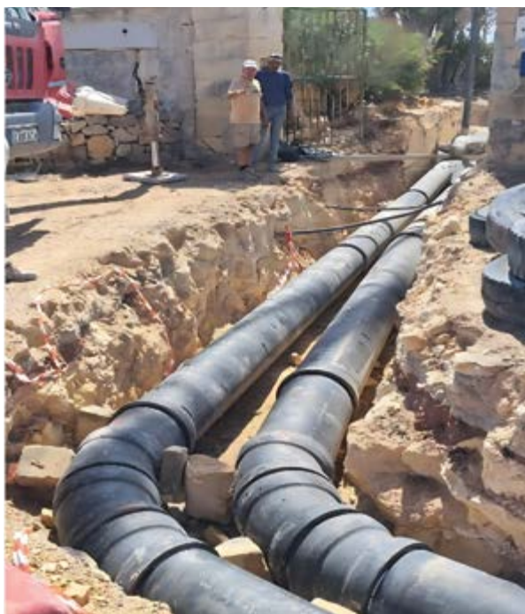
Figure 31 Works showing the connection of the two reservoirs
