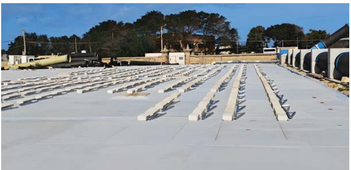
Figure 79 Extensive refurbishment at Ta' Qali Group of Reservoirs
