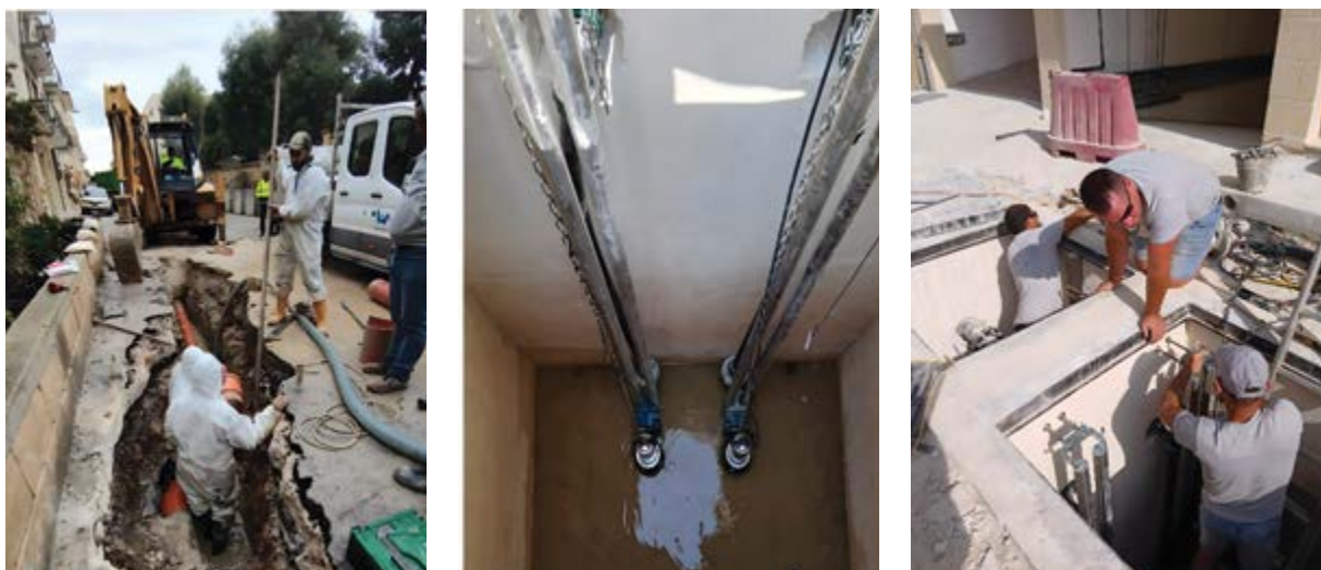
Figure 35 Sewer replacements and new pumping stations
