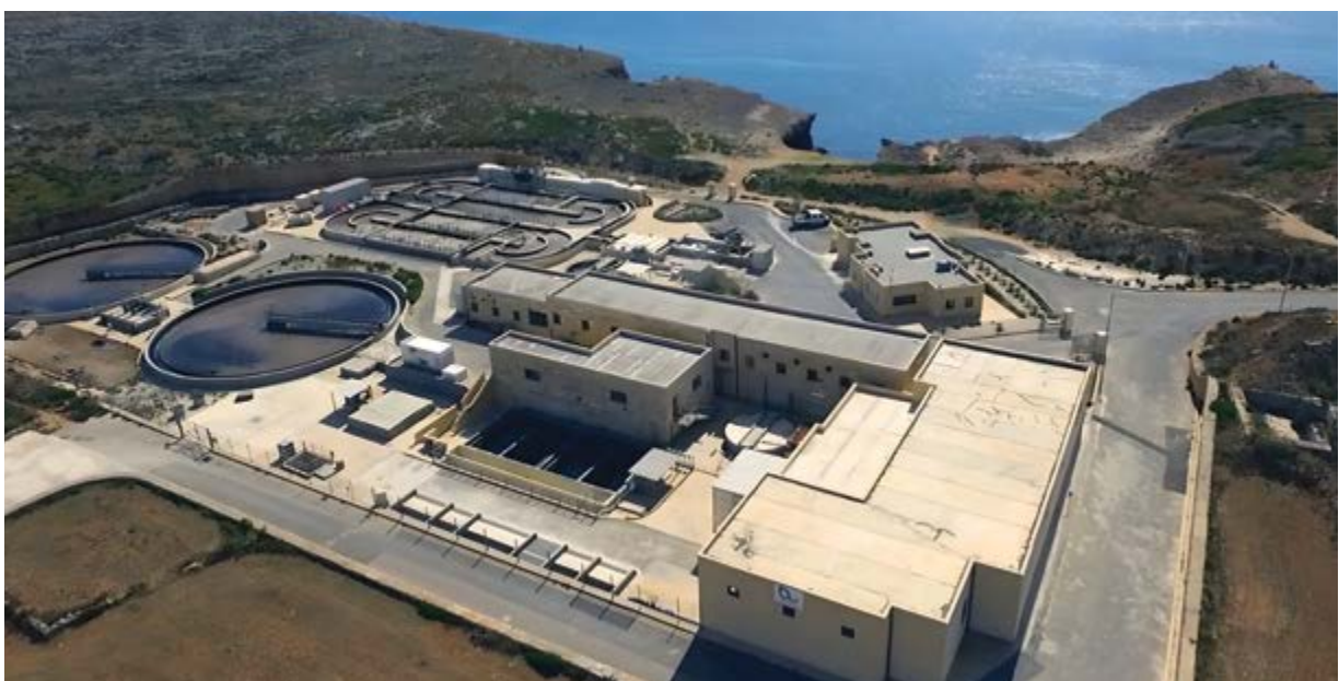
Figure 50 WSC contracted the upgrade of the Malta North WWTP
