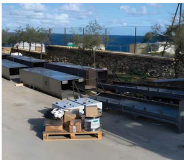
Figure 48 Installation of new coarse screens completed
