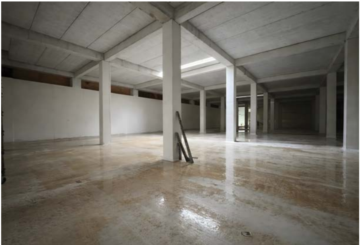
Figure 42 Naxxar reservoir refurbishment
