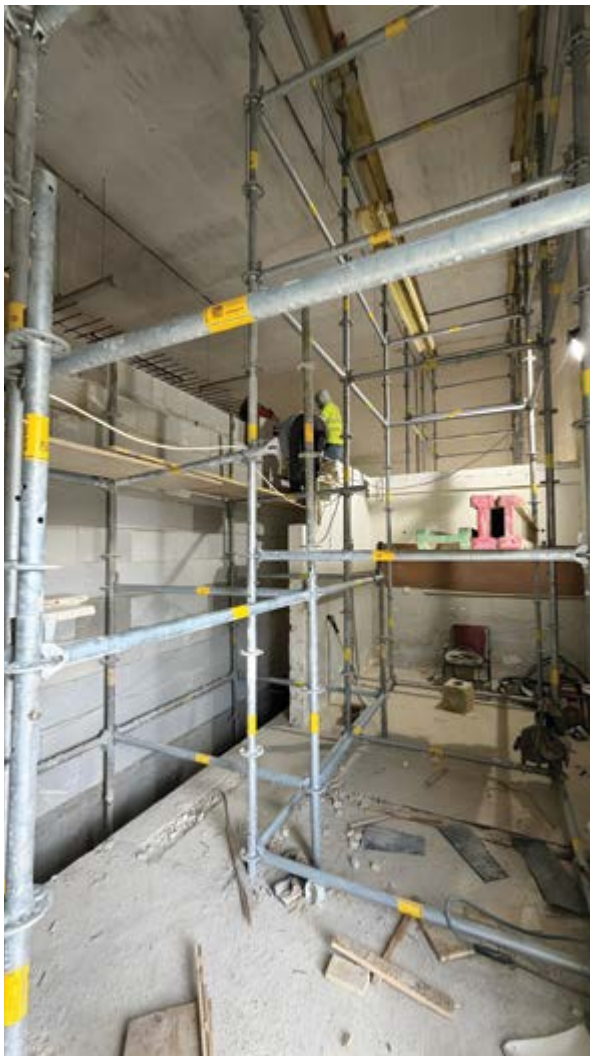
Figure 83 Extension of transformer room and construction of new switchgear room at Lapsi RO plant
