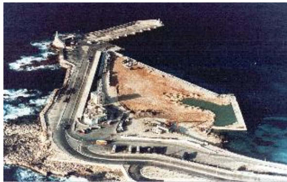
Figure 8-3: Cirkewwa Ferry Terminal reclamation (Source: MMA)
