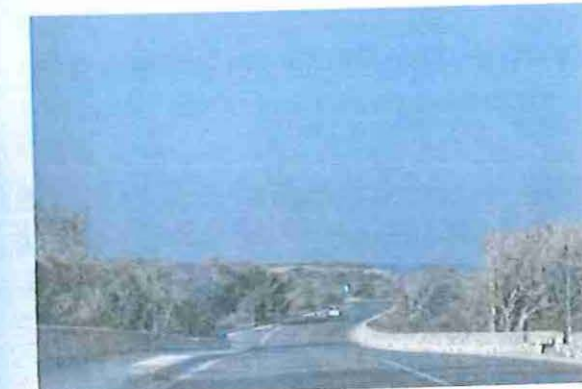
East to West Road in the North Coast of Malta Island
